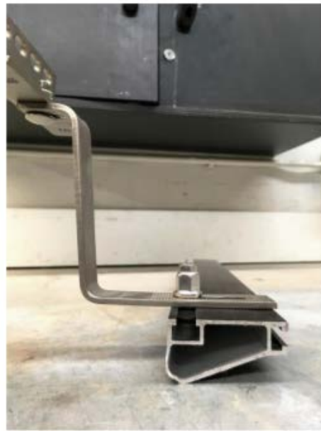
Figure B2d. Side view of connection
