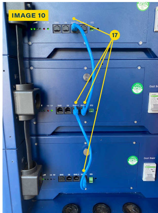
17 USE INCLUDED NETWORK CABLES TO DAISY CHAIN BATTERIES FROM PS485-2 PORTS
