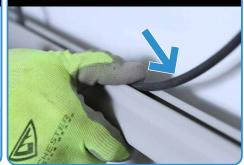
Install Panels: As each panel is secured to racking, connect cables and push any remaining slack into PVshield.
