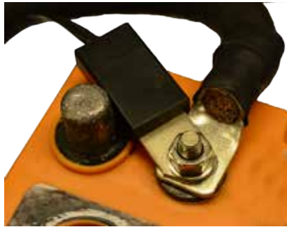
Fig 2.5(b) Temperature Sensor Installation
